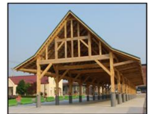
Alabama's Largest Timber Frame Structure
